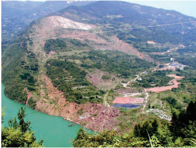
Figure 21.12 A massive rock block landslide which occurred on 13 July 2003, in Qian-jiang-ping, Zigui County, blocking the Qinggan River, 3 km from the river mouth discharging into the Yangtze, and about 20 km upstream from the Three Gorges Dam
