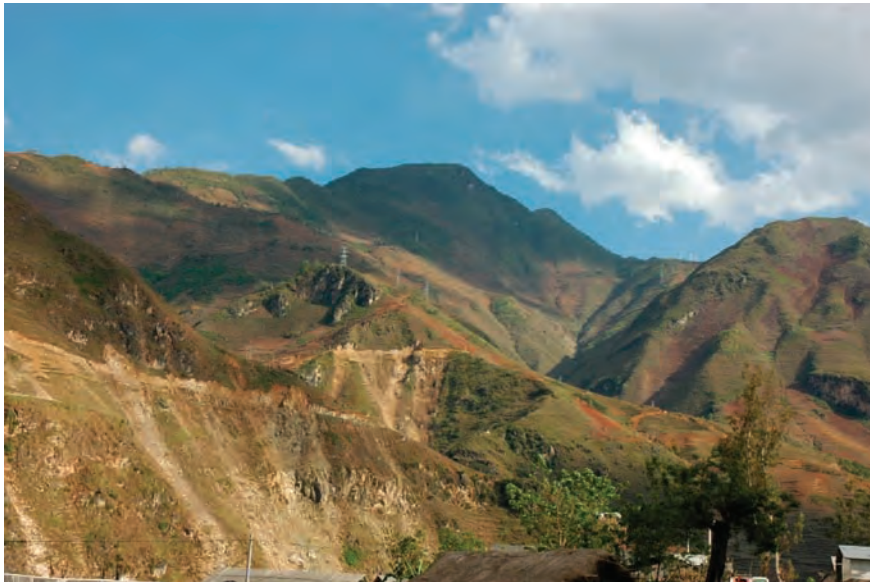
Figure 21.9 Field photo taken in April 2006 on the road along the Nujiang Valley. The picture shows the destruction of vegetation coverage by road cutting and excessive cultivation
